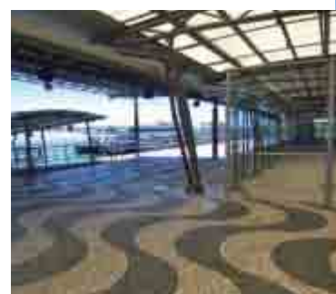
Terminal Roda-Ferro-Fluvial, Portugal
